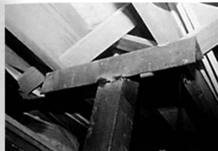
Floors beneath rubbleized portions of buildings can be braced to afford camouflage and protection.
