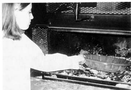
Common fireplace inserts or stoves can be converted into "spark heaters" by using a large pan full of fuel oil. Fumes from the oil are burned to produce low-grade, economical heat.
